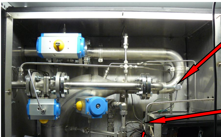
Heater with temperature sensor
