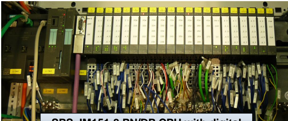
SPS, IM151-8 PN/DP CPU with digital and analogue cards
